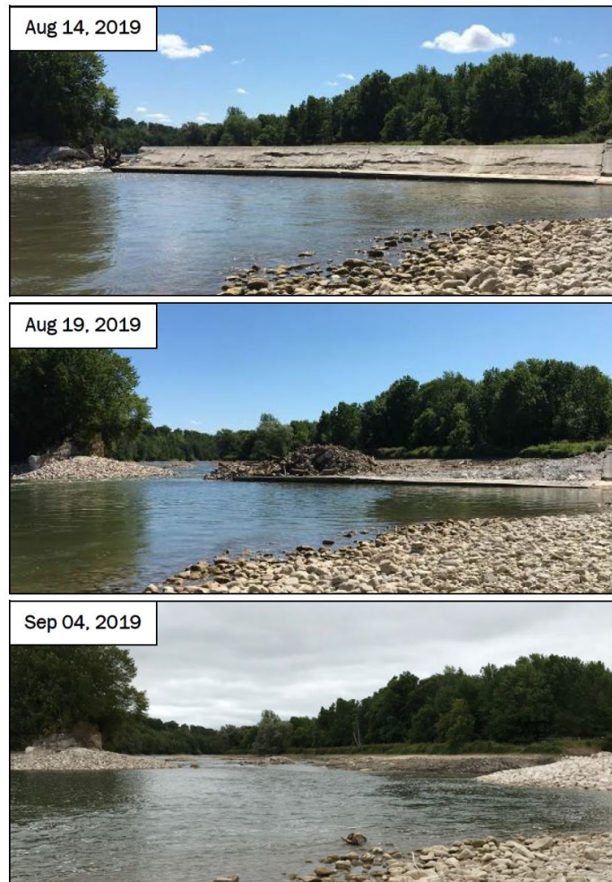
Figure 57 - Truax Dam, Walkerton, Ontario.
