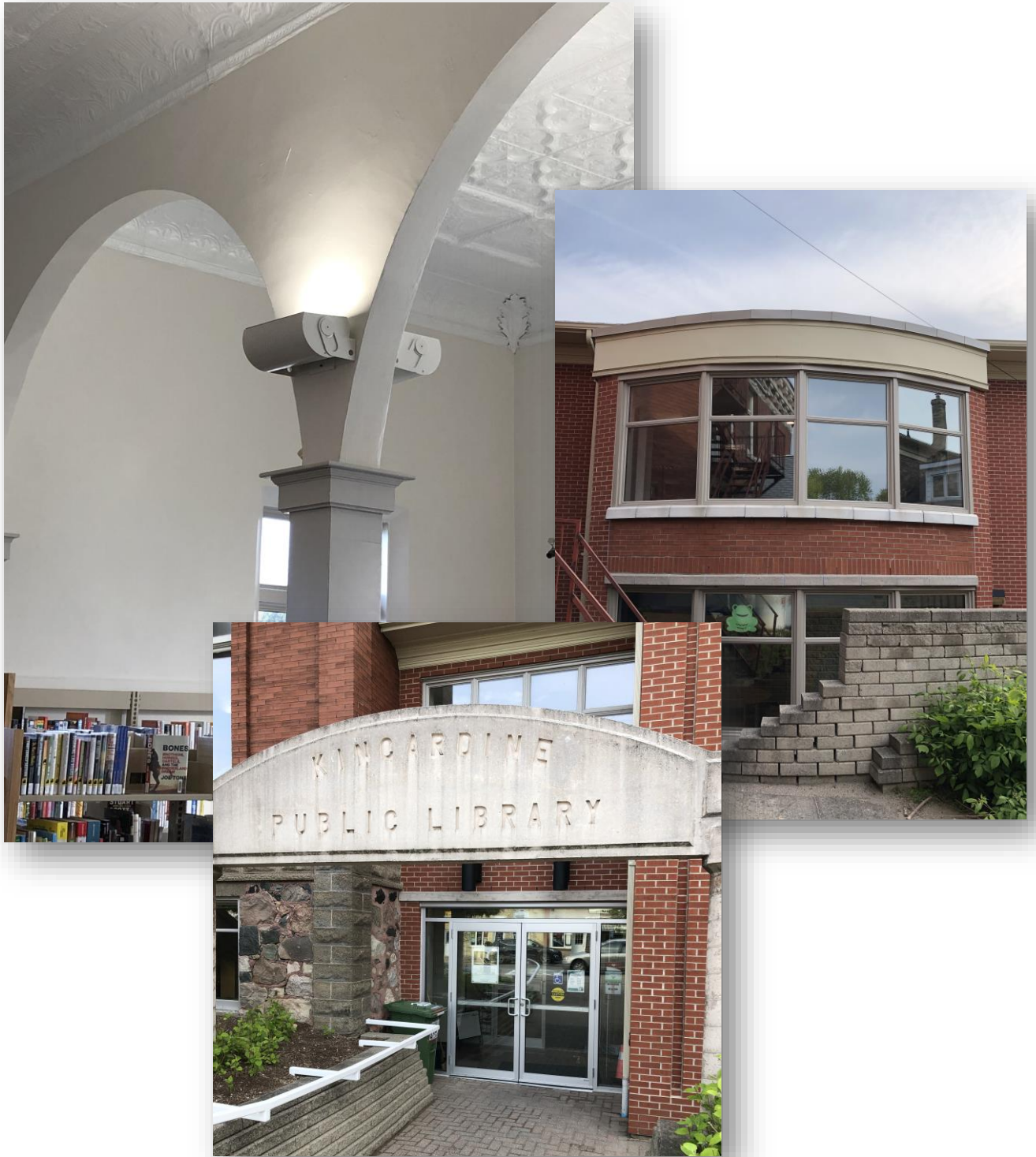
Figure 4: Energy efficient LED lighting upgrades, new windows and doors at the Kincardine Library
