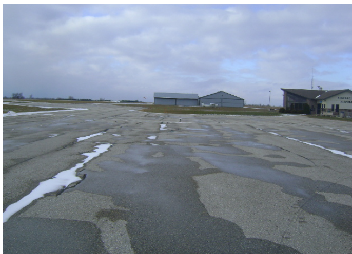
Typical Pavement Conditions on Apron I
