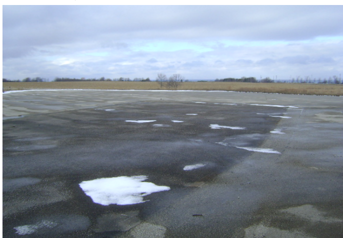
Typical Pavement Conditions on Apron II
