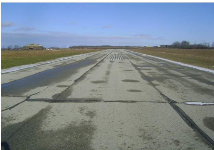
Typical Pavement Conditions on Runway 05-23
