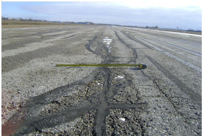
Typical Pavement Conditions on Runway 13-31
