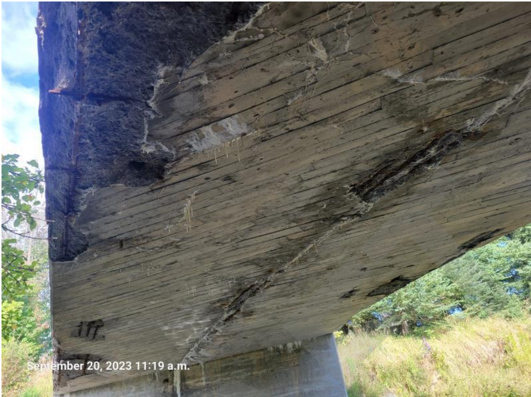
3-Soffit From East Abutment
