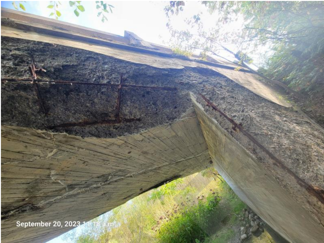
5-Southeast Wingwall and South Deck Edge
