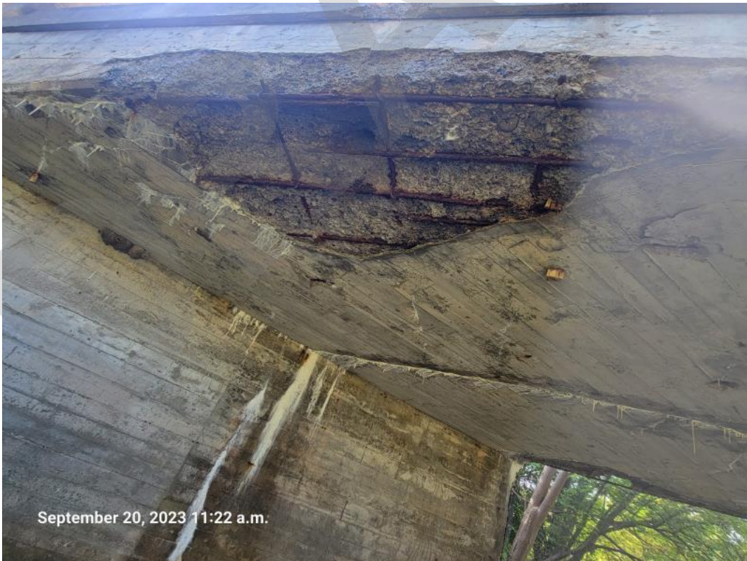
8-Soffit at Northeast Drain
