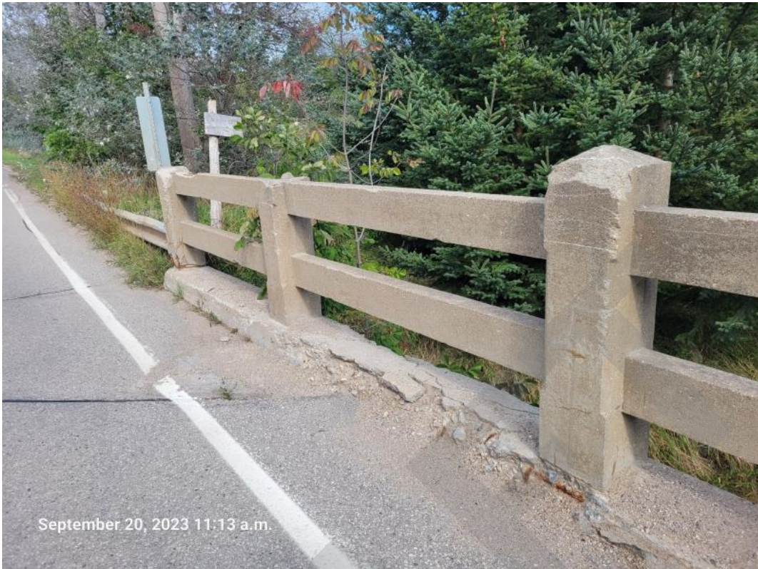
Northwest Railing End
