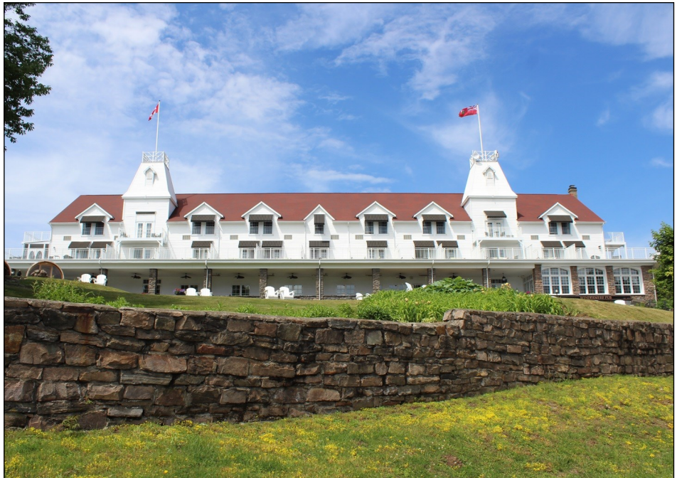
Windermere House on Lake Rosseau was restored and renovated by architect and designer David Gillett. (Photo by James Forrester, Selwyn Twp. Heritage Committee)
