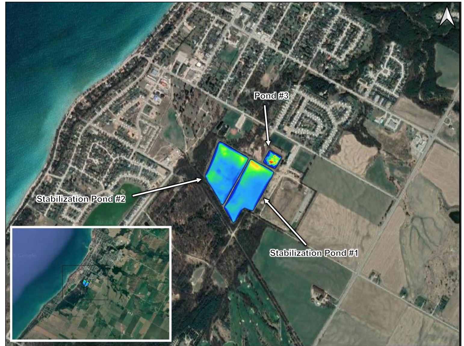
Figure 1 Kincardine, ON Wastewater Lagoon overview
