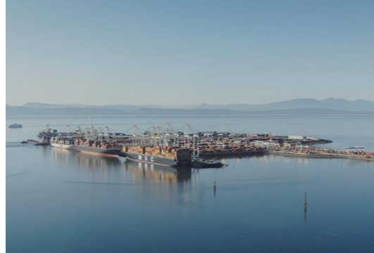
Deltaport Fourth Berth Project
