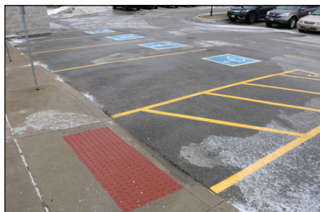
Accessible parking spaces with access aisle and curb ramp, City of London.
