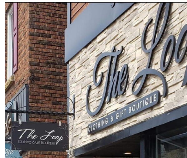
Stone veneer façade
