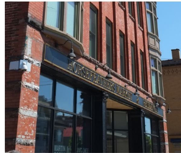
Painted transom and window details with exposed brick columns
