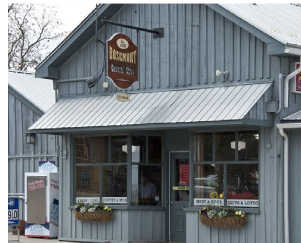
Board and batten exterior
