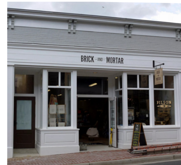
Painted brick, base and transom, and cornice detailing
