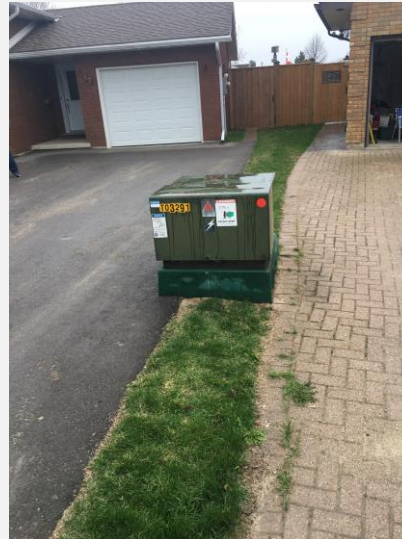
Kincardine Underground Rebuild
