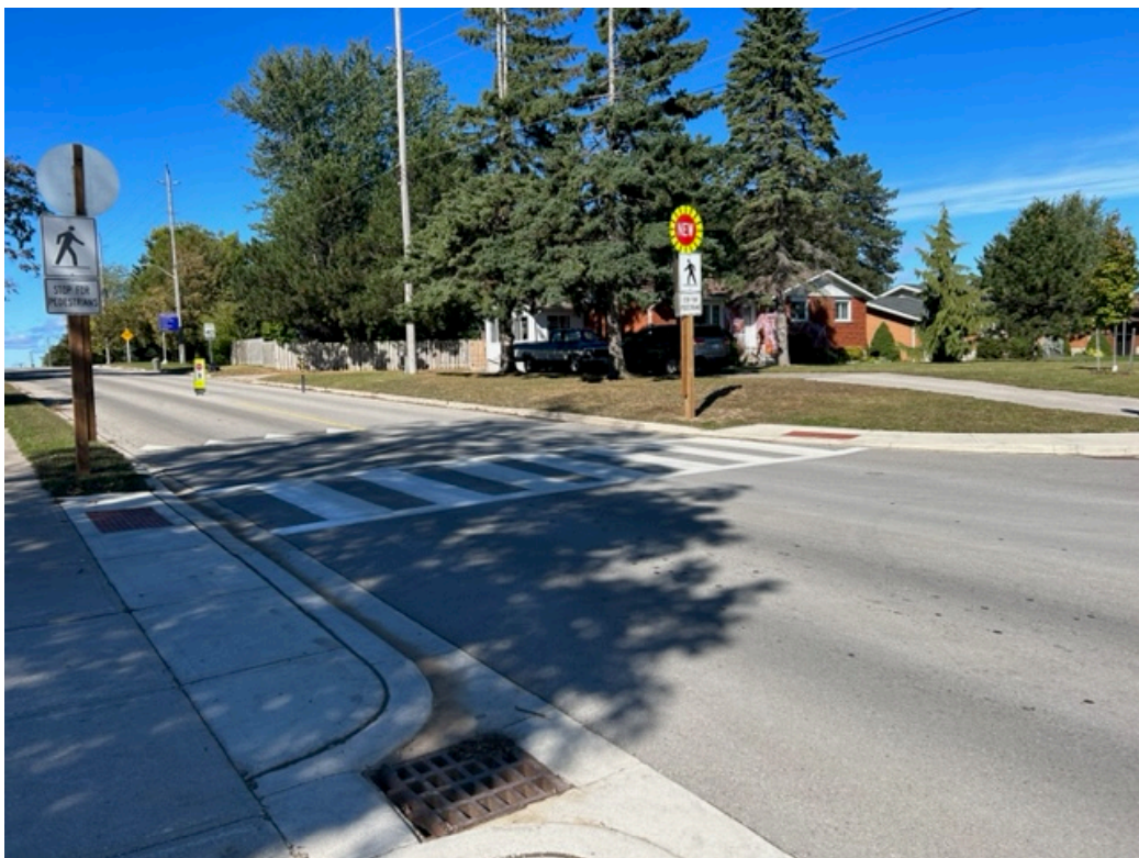
Newly installed crosswalk at Bruce Ave & Princess Street
