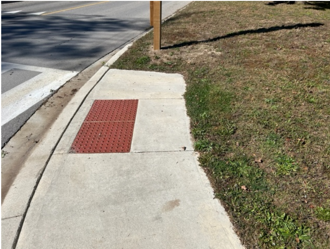
This crosswalk is at station beach It to does not meet the AODA It does not have the audible
