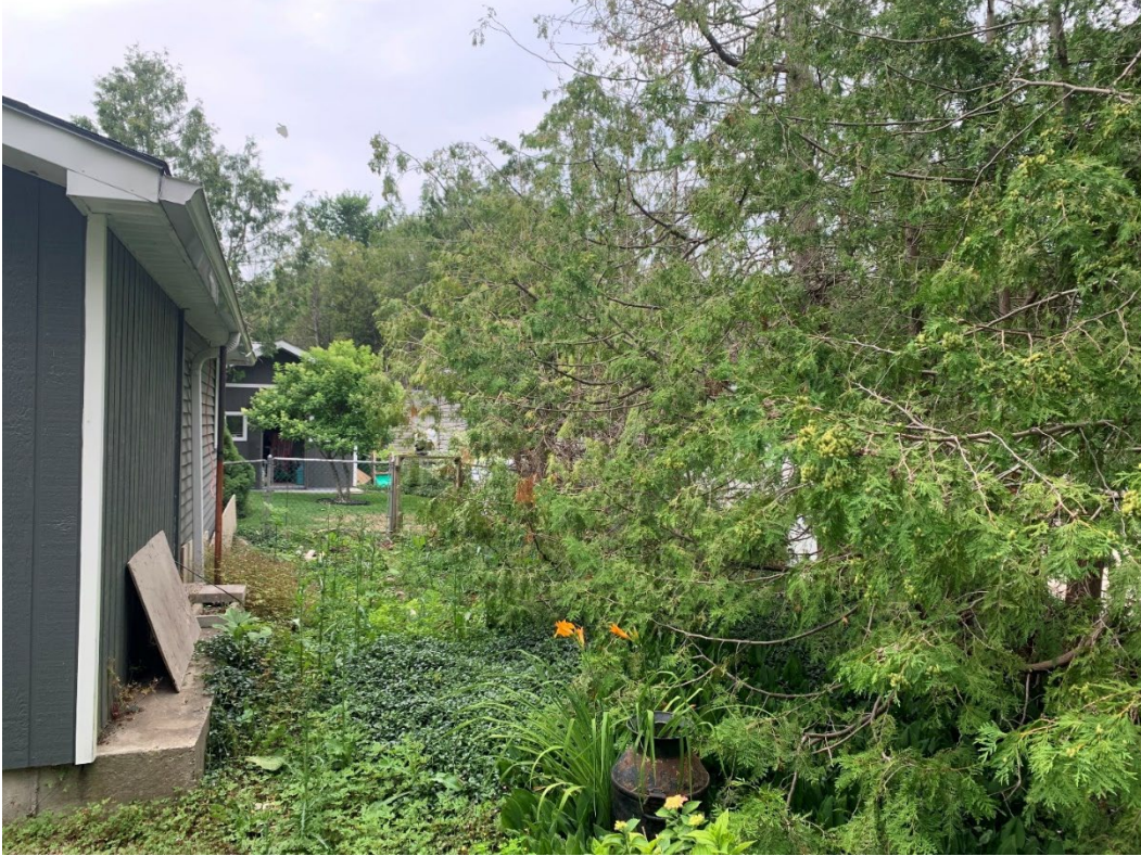
Image of Existing Structure
