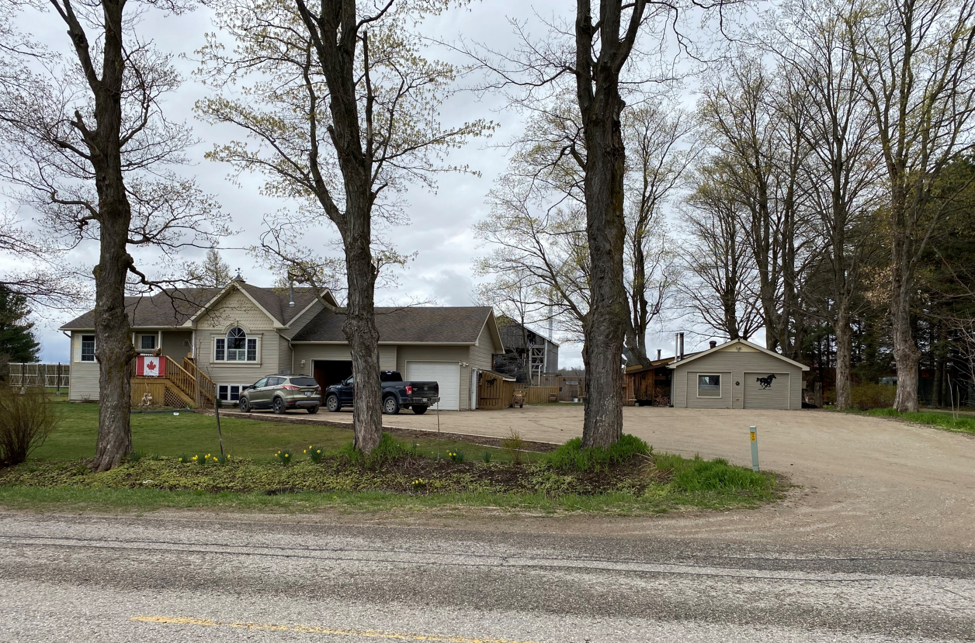
Front View - Looking from Concession 2
